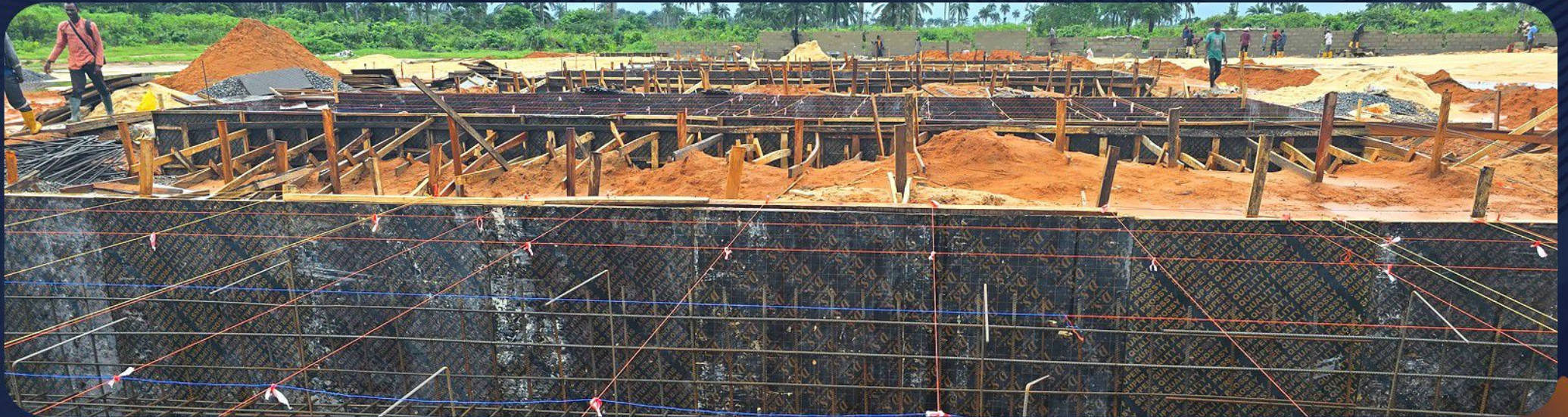
The commencement of 4 Compressor foundations
