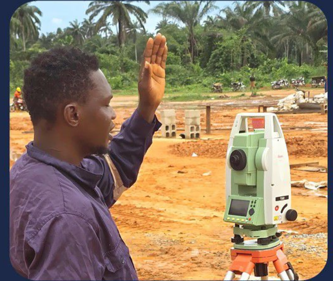
Site surveyor(s) setting out horizontal and vertical alignment of bolt positions
