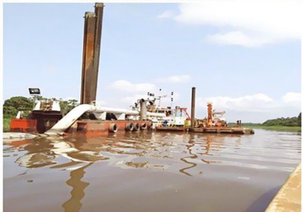
Dredger with a Multicat at Ovhor Field for capital Location Dredging
