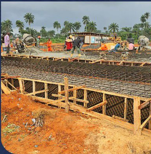
Reinforcement works for module foundation works
