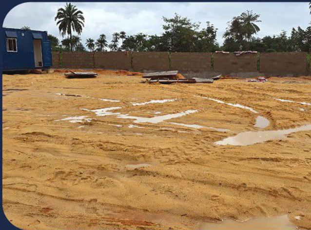
Concrete wall fence construction at Phoenix Kwale Gas
