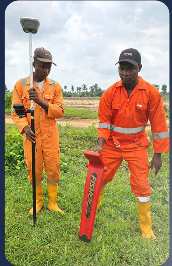
Osбето team carrying out asbuilt survey for pipeline construction
