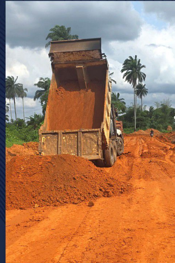
Sand offload at site as Road construction for PIDL continues
