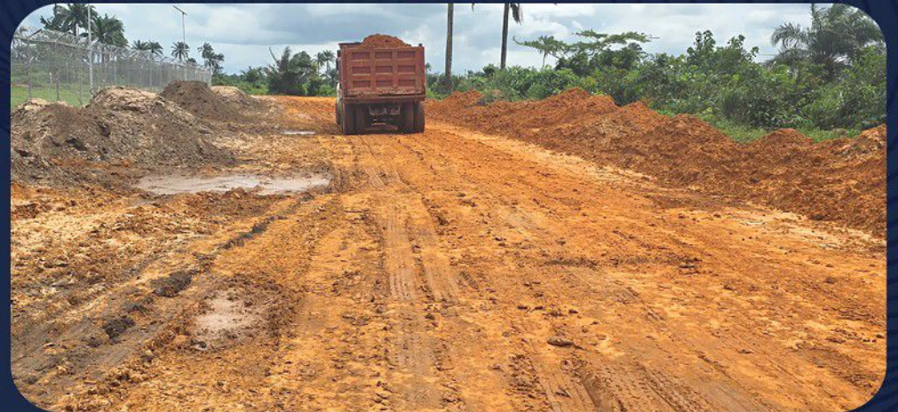
Location Road Construction
