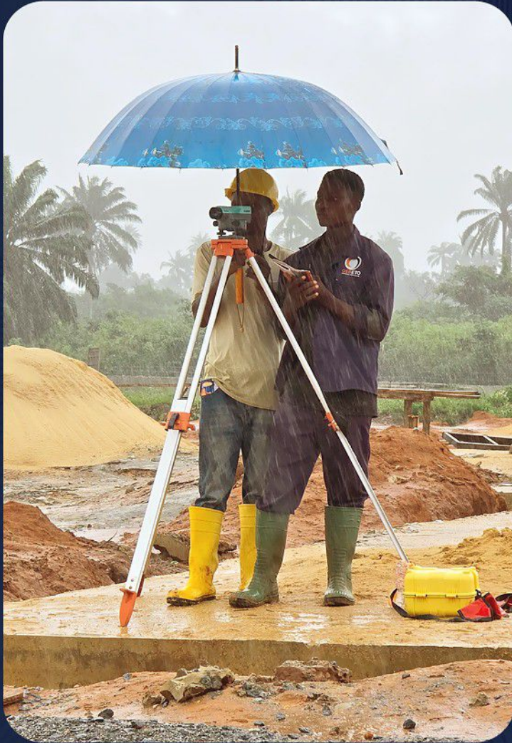
Osbito survey team working on site
