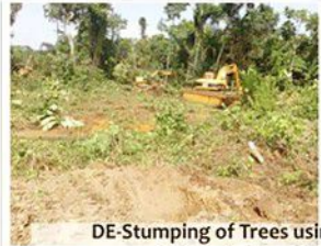
DE-Stumping of Trees using Drypants Equipments at Ovhor field capital Dredging Location
