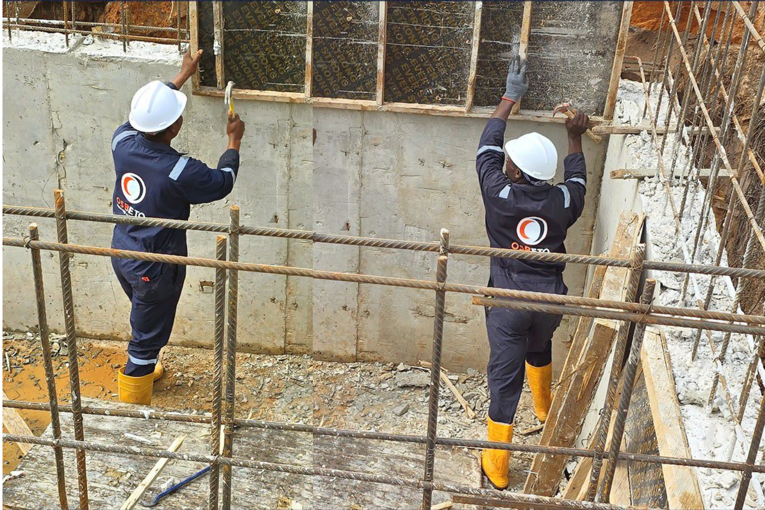
Building of Closed Drain
