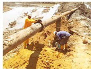
Shoreline coupling at the Dredging Location
