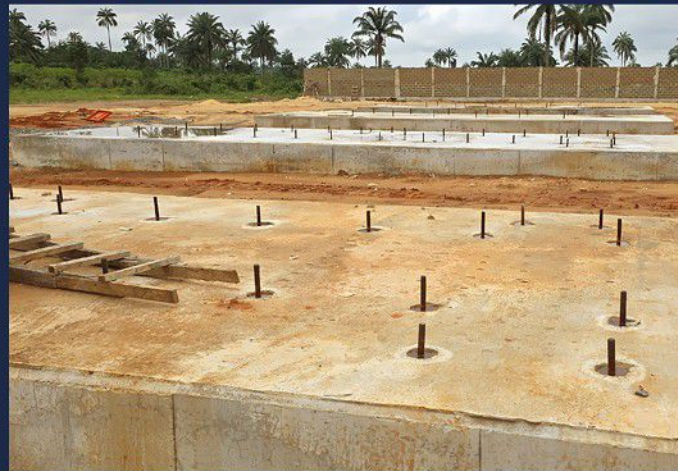
Gas compressor foundation upon completion
