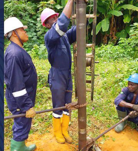
Osбето team carrying out Geotechnical survey for Xenergi Limited at Kwale Free Trade Zone
