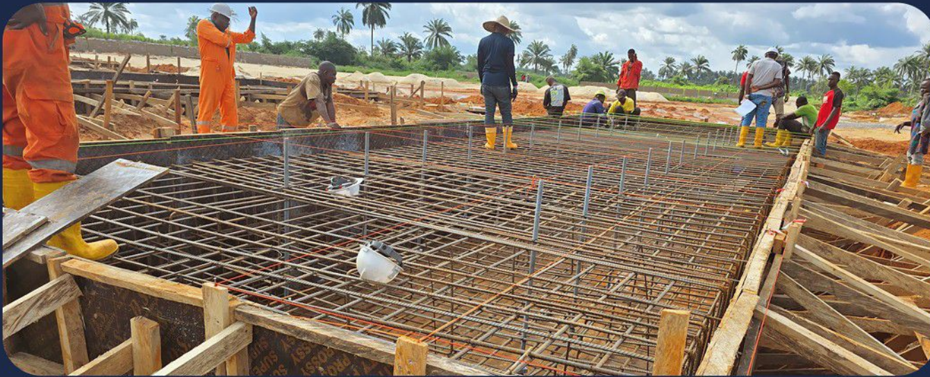
Reinforcement phase of the compressor foundation
