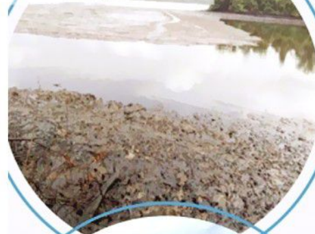
Siltation Sweeping of Ubefan Well 2 & 4, Slot and Access, Odidi
