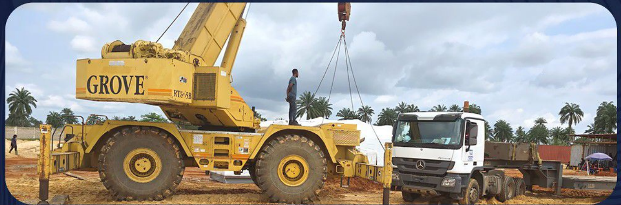
Facility installation process at one of our sites
