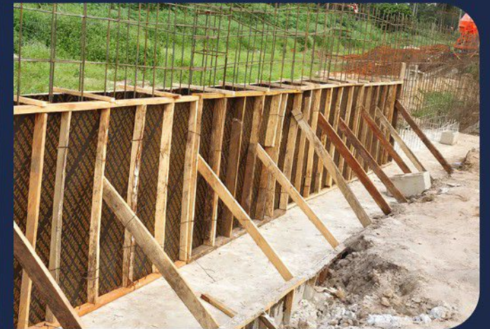
Concrete wall fence formation on site
