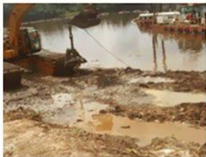
Dredging Operation and Anchor Positioning
