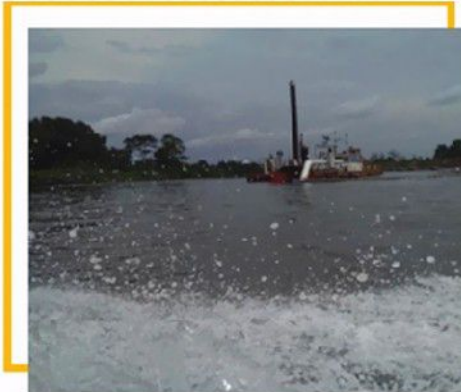
Sweeping Near Completion
