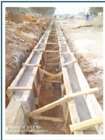
Drainage Construction at Iguelaba, Edo State
