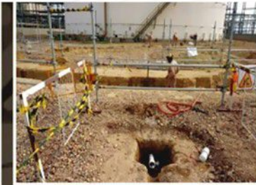
TANK FARM FOUNDATION
