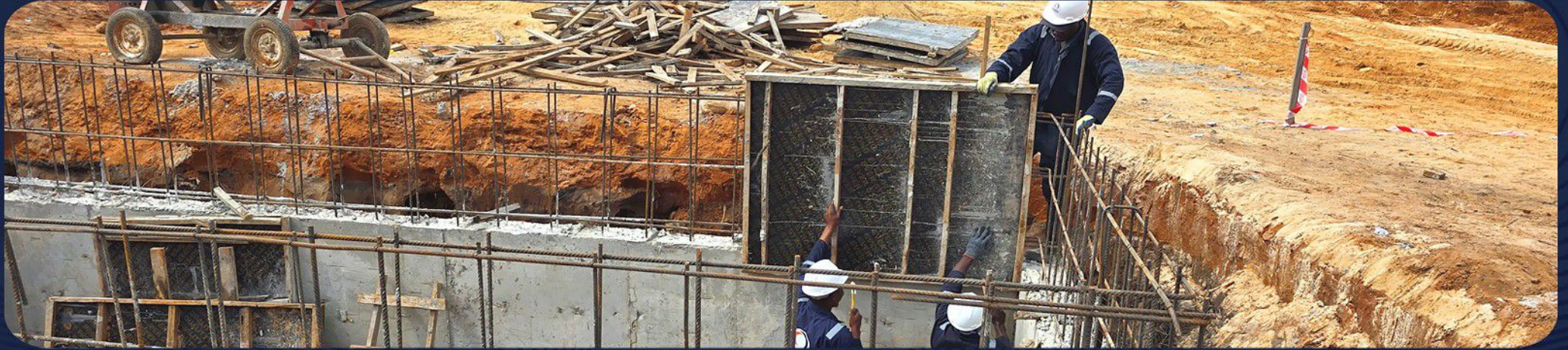
Building of Closed Drain(s)
