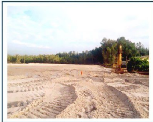
Reclamation Site of New Diebiri Batan, Delta State
