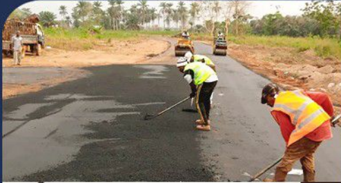
A Road Construction Project
